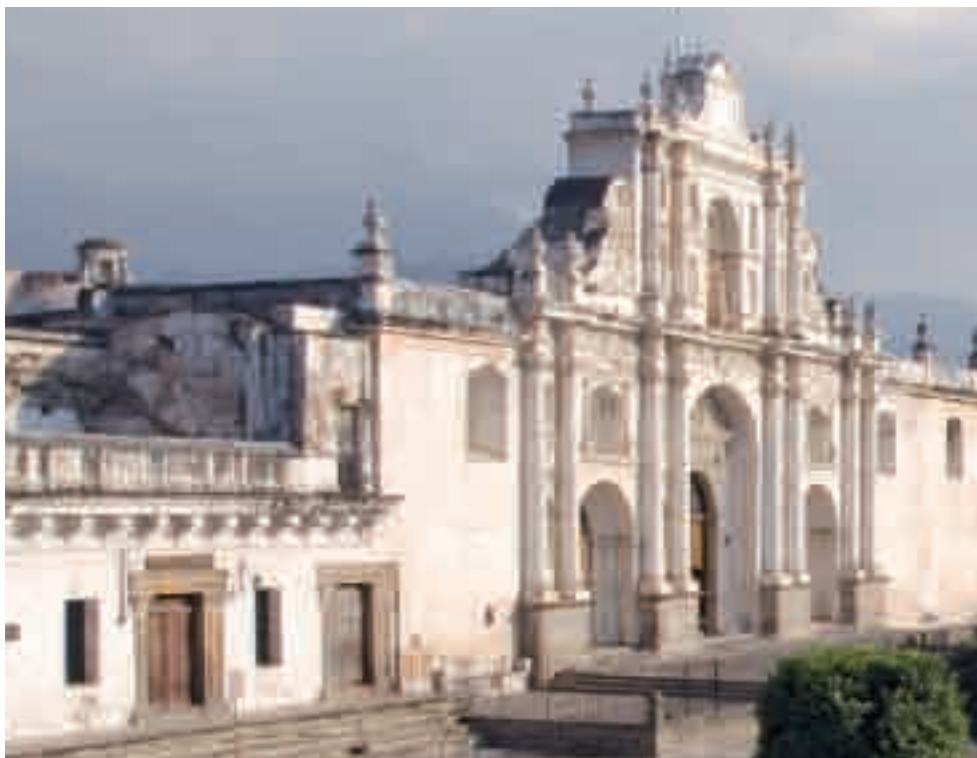
Park Central, Antigua - Guatemala
