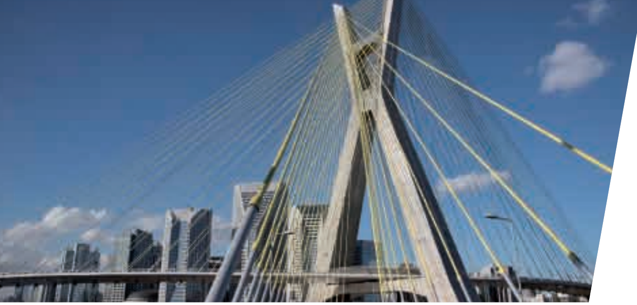
Bridge Octavio Frias de Oliveira, Saint Paul - Brazil
